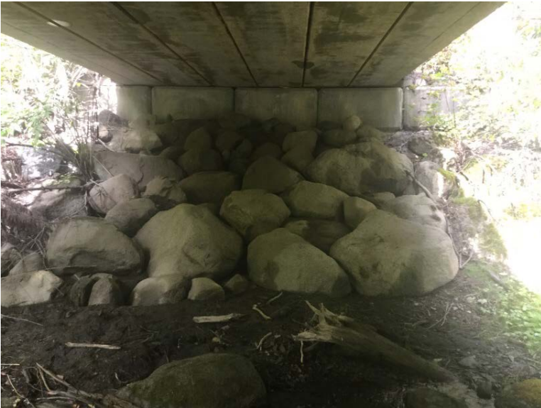
Left Bank Abutment when facing downstream
