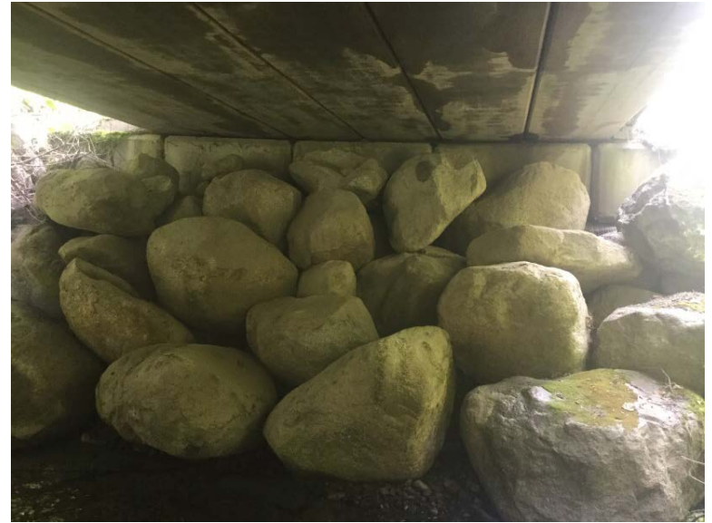
Right Bank Abutment when facing downstream
